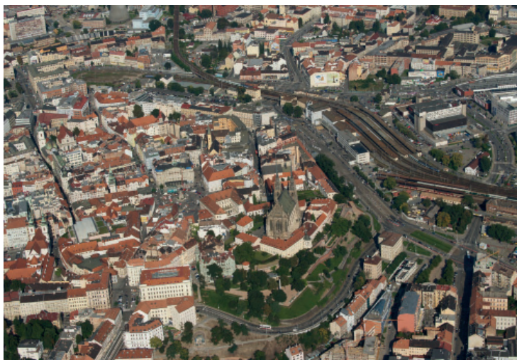
Brno – air shot onto historical part
